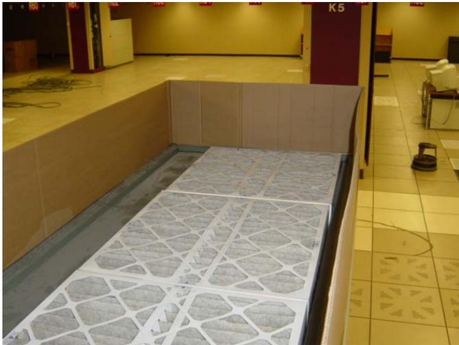
Fig. 3. Cardboard box installed on the top of the A/C unit (filters are covering the air intake of the A/C unit)
